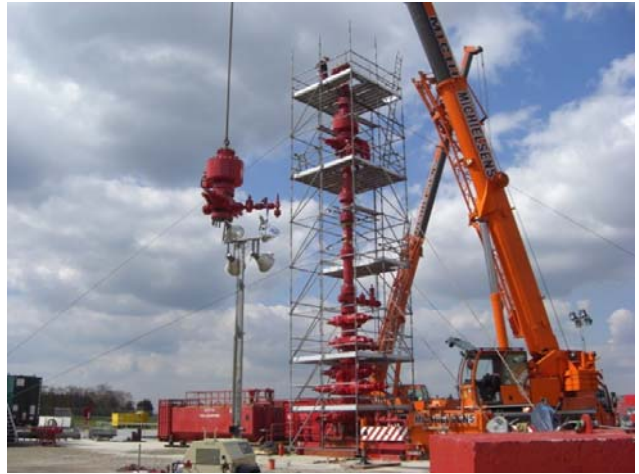
Figure 6 – Halliburton HWO – Stack-up
